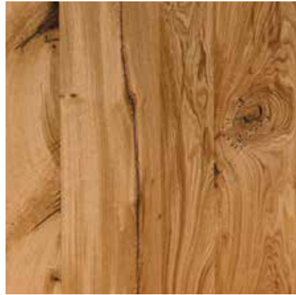
BEAM OAK CRACKS
