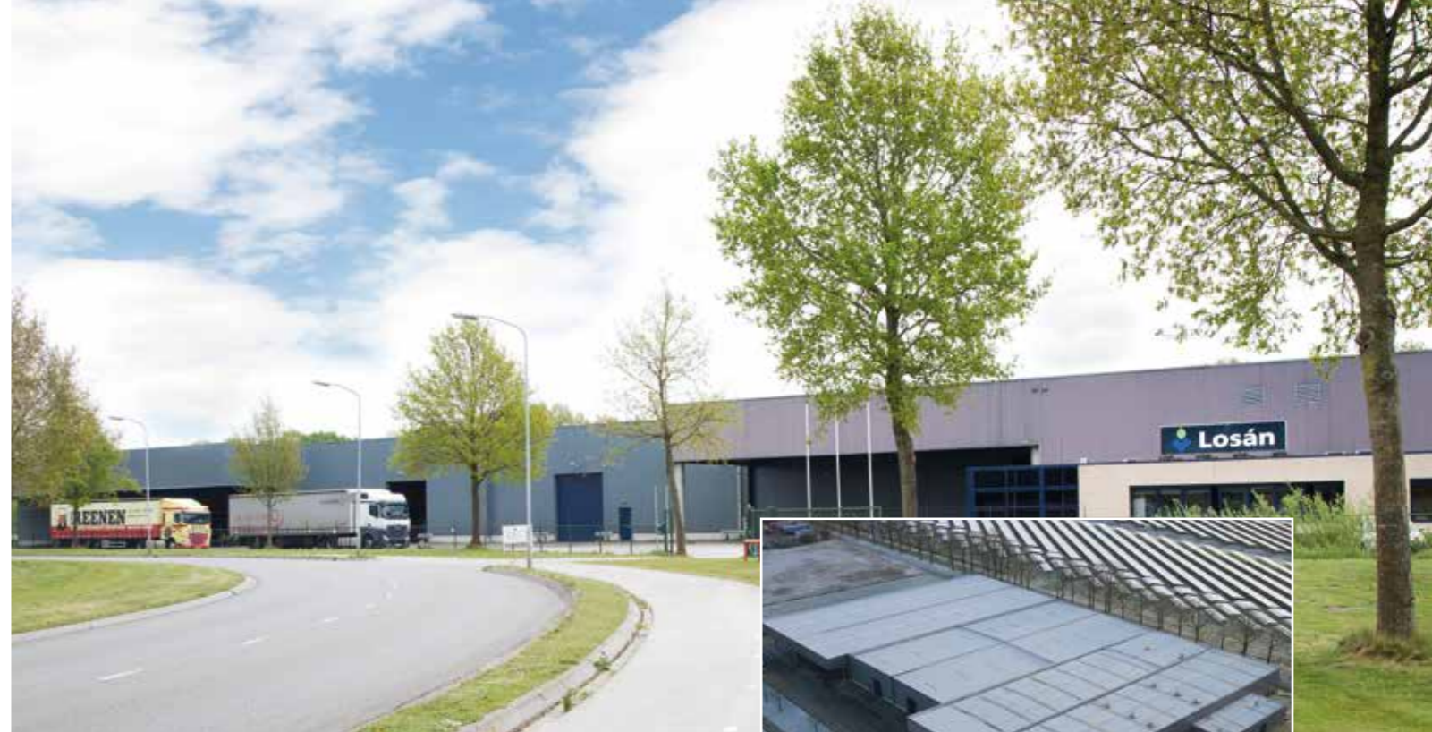
Emmen, office building
